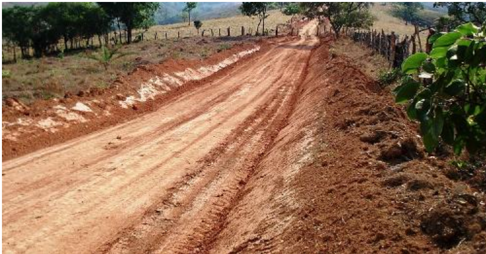
Figure 3: Dirt Road made of sand, gravel, mountain soil and cement
