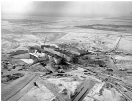
The early construction of Launch Pad 39A
