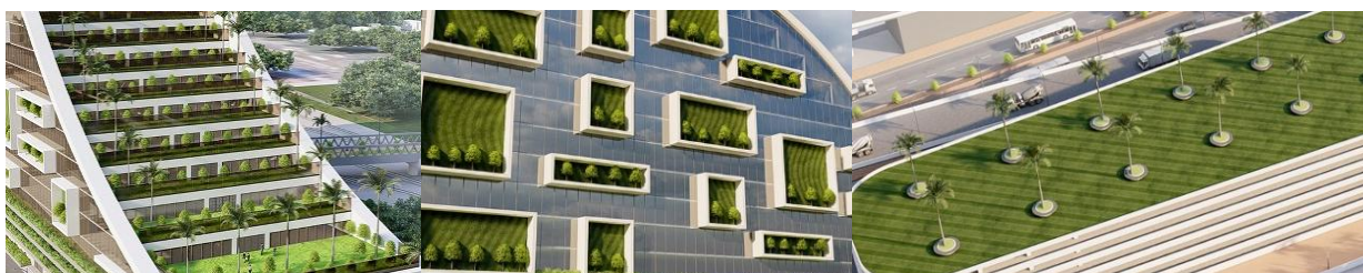
Figure 4. The green roof and green wall.
