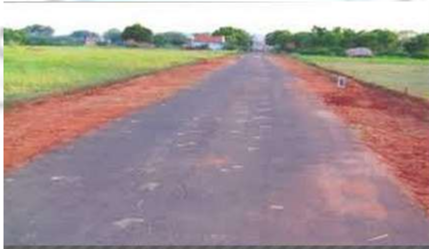
Figure 3: Widening of rural roads
