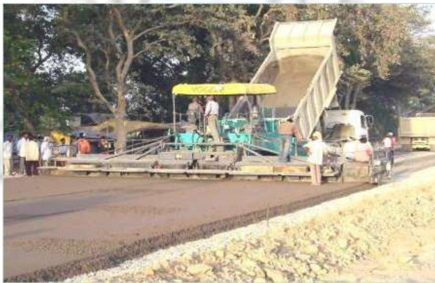
Fig. 2: Laying of DLC of the recycled concrete
