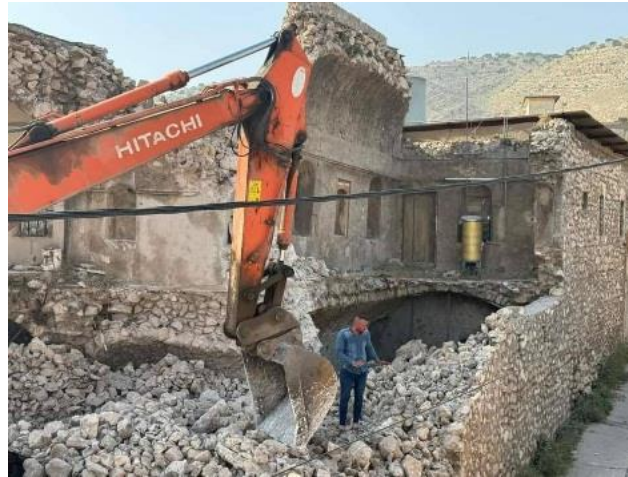
Figure 4. Heritage demolition for new construction.
