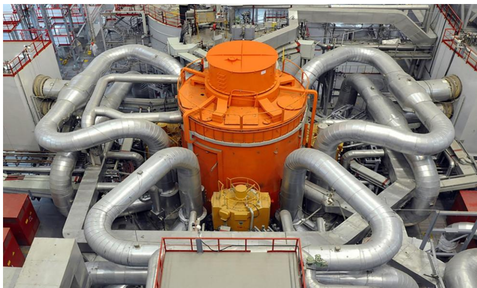
Figure 5 - The BN-800 reactor at the Belyarsk Power Station in Russia Source: IAEA (2020)
