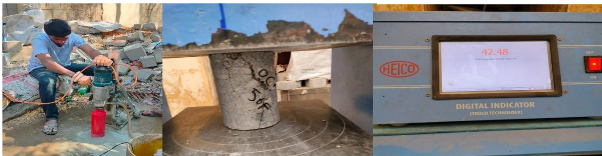
Figure 5. Concrete Core Test
