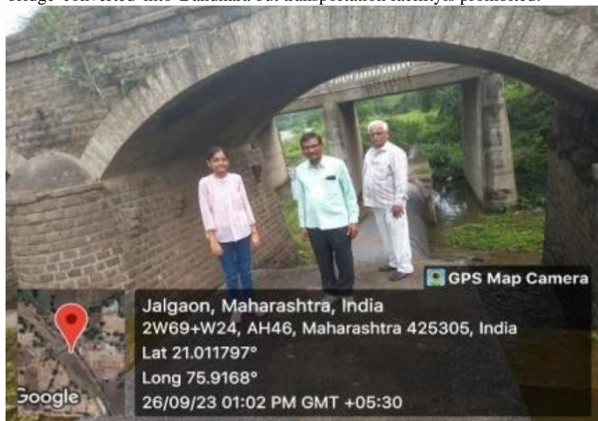
Fig No. 5 Varangaon Site Visit
