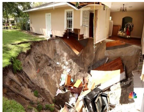
Fig 4 (Foundation damage due to Sinkhole)
