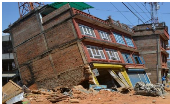
Fig 1 ( Foundation failure caused the collapse of this building in Chautara Sindhupalchowk )
