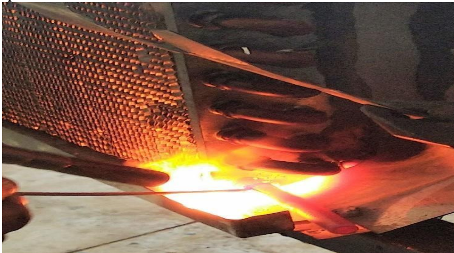
Fig 18 Our Project While Fabrication
